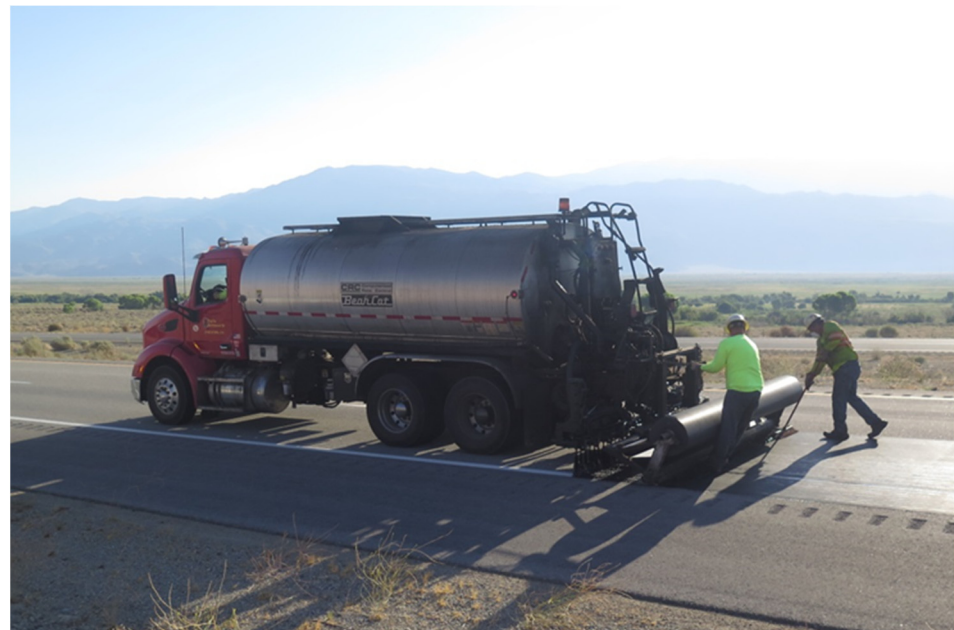
Figure 3. Distributor truck equipped with fabric bracket to apply PG 70-10 binder and paving mat or PRF.
