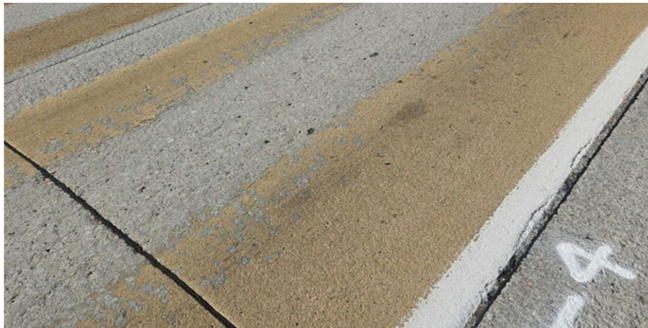
Figure 3. Experimental Bauxite Material with Underlying Concrete Visible
